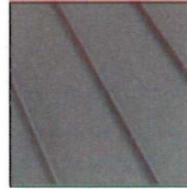
4. STANDING SEAM METAL ROOF
