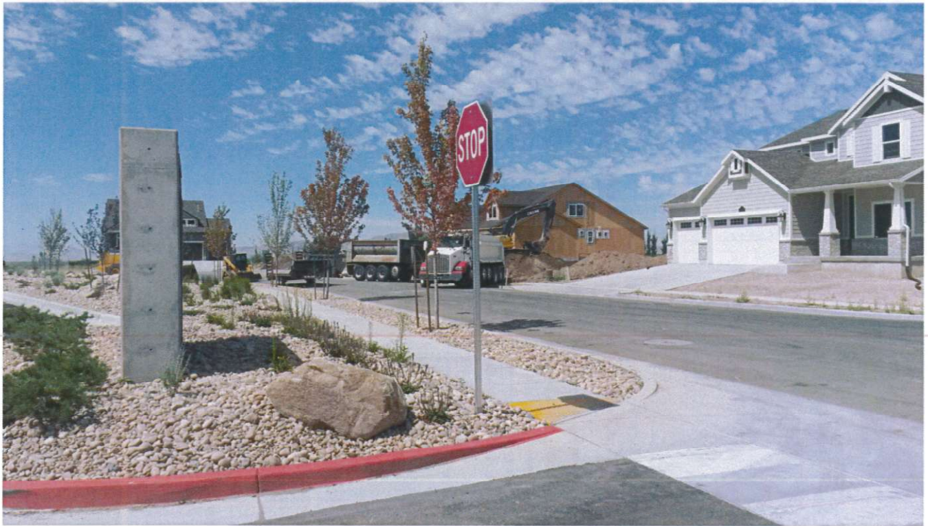
Photo 1: View of the intersection from the northbound lane, looking south. The stop sign is visible on the right side of the road. The excavator is working on the dirt mound in the background.
