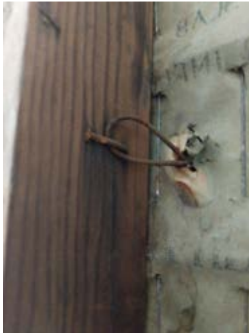
Photograph 12 – Wire anchorage observed between stone wall and wood stud interior wall
