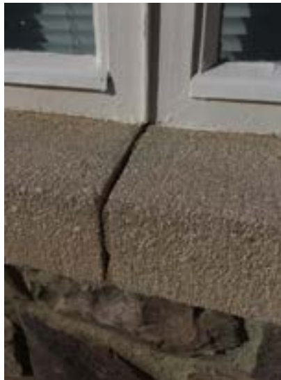
Original steel window and cast concrete sill.
