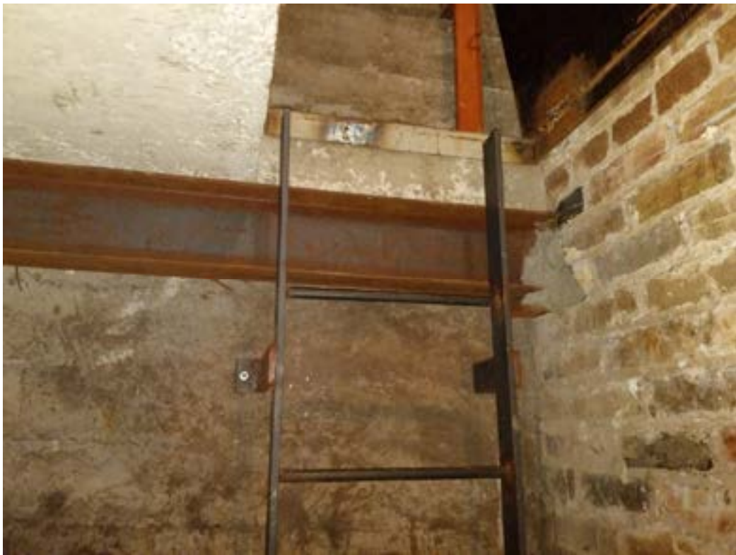
Photograph 14 – Underside of coal storage, six inch concrete slab with steel wide flange support beams
