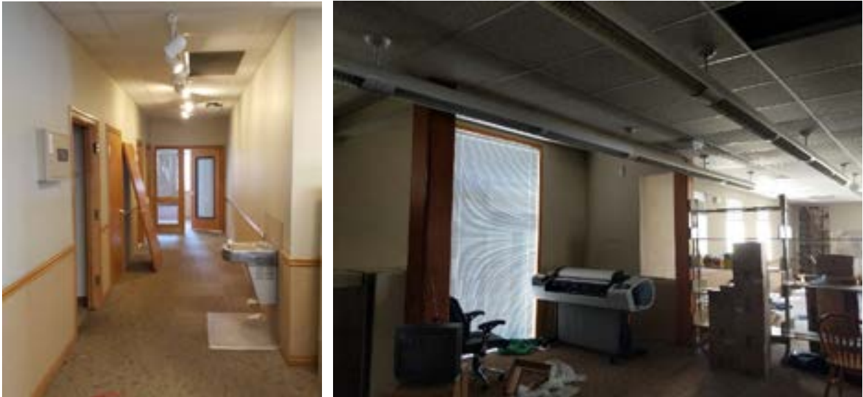
Photograph 9 – Interior Bearing Systems. Left: Wood stud wall running North-South on East side of building, Right: Beam – header configuration on North-West side of building
