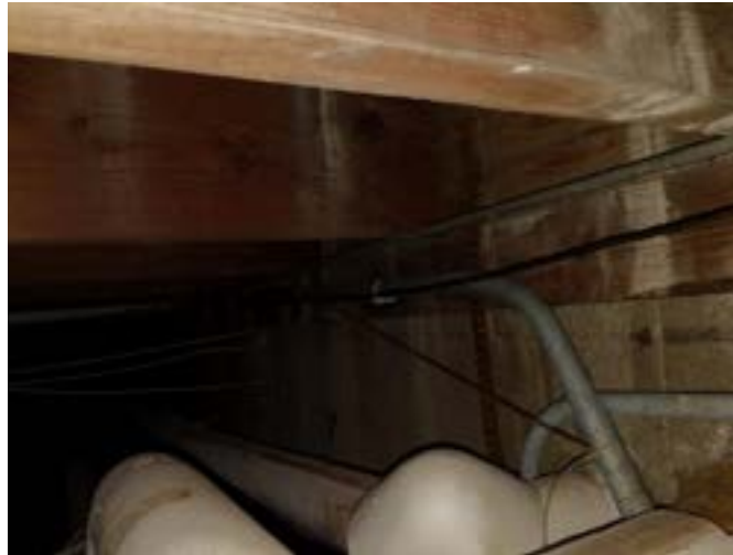
Photograph 16 – 2x4 ledger supporting floor joists.
