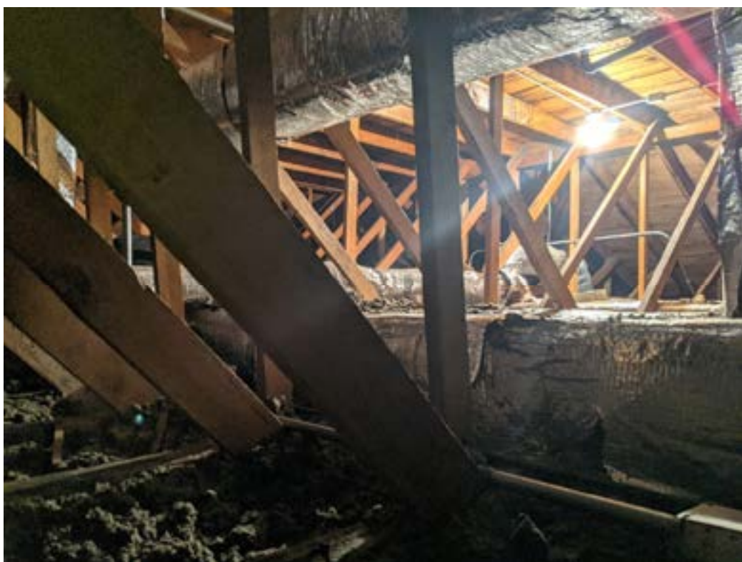
Photograph 5 – Roof truss framing viewed from attic access
