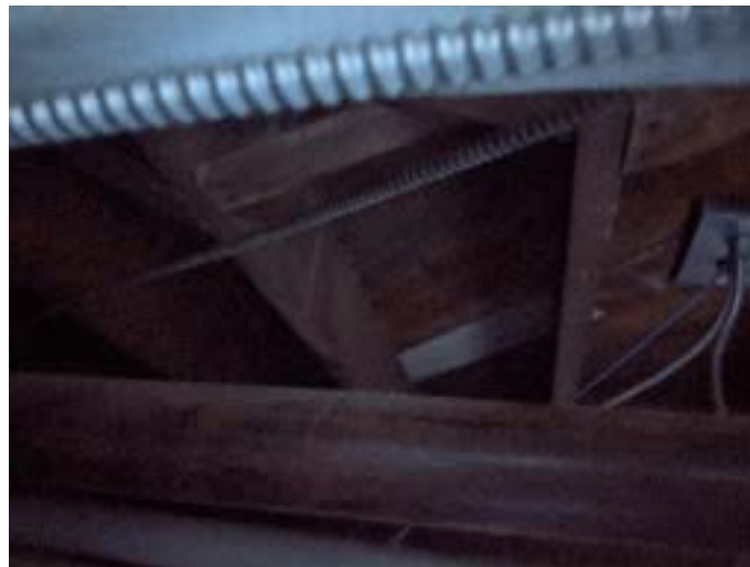
Photograph 17 – Diagonal 1x floor sheathing
