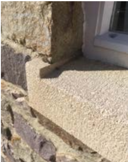
Original steel window and cast concrete sill.
