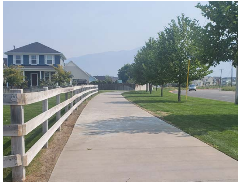
Existing pathway along 200 North in Kaysville.
