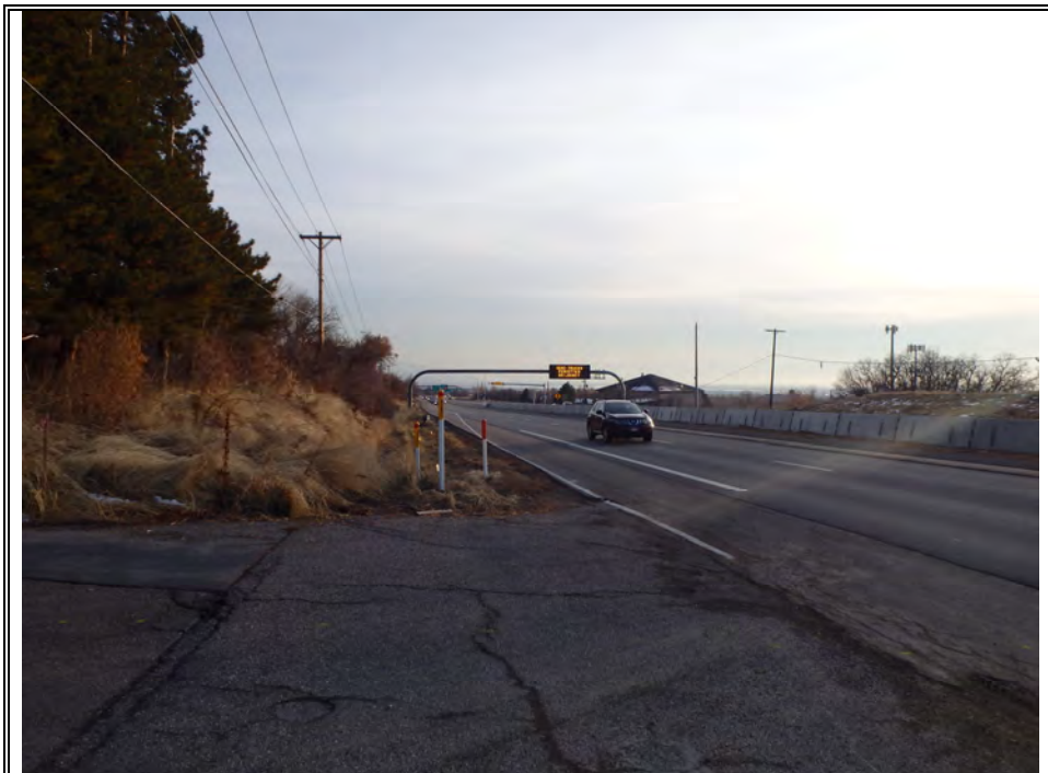
Highway 89 Looking South
