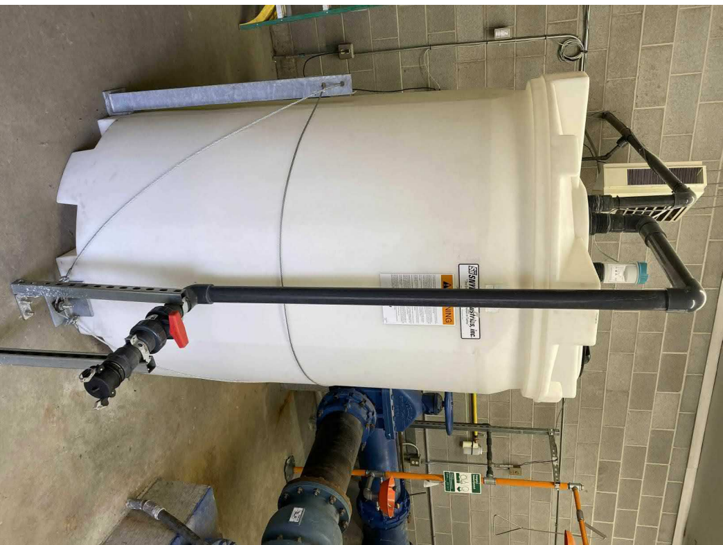
DETAIL - CHLORINATION TANK
