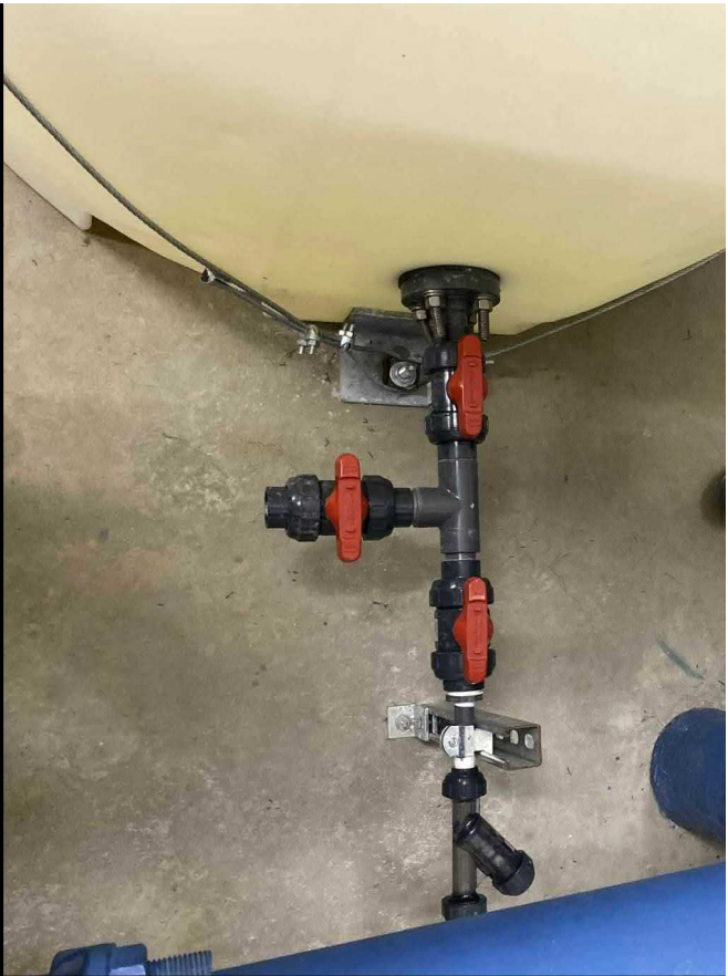
DETAIL - CHLORINATION TANK - OUTLET PIPE
