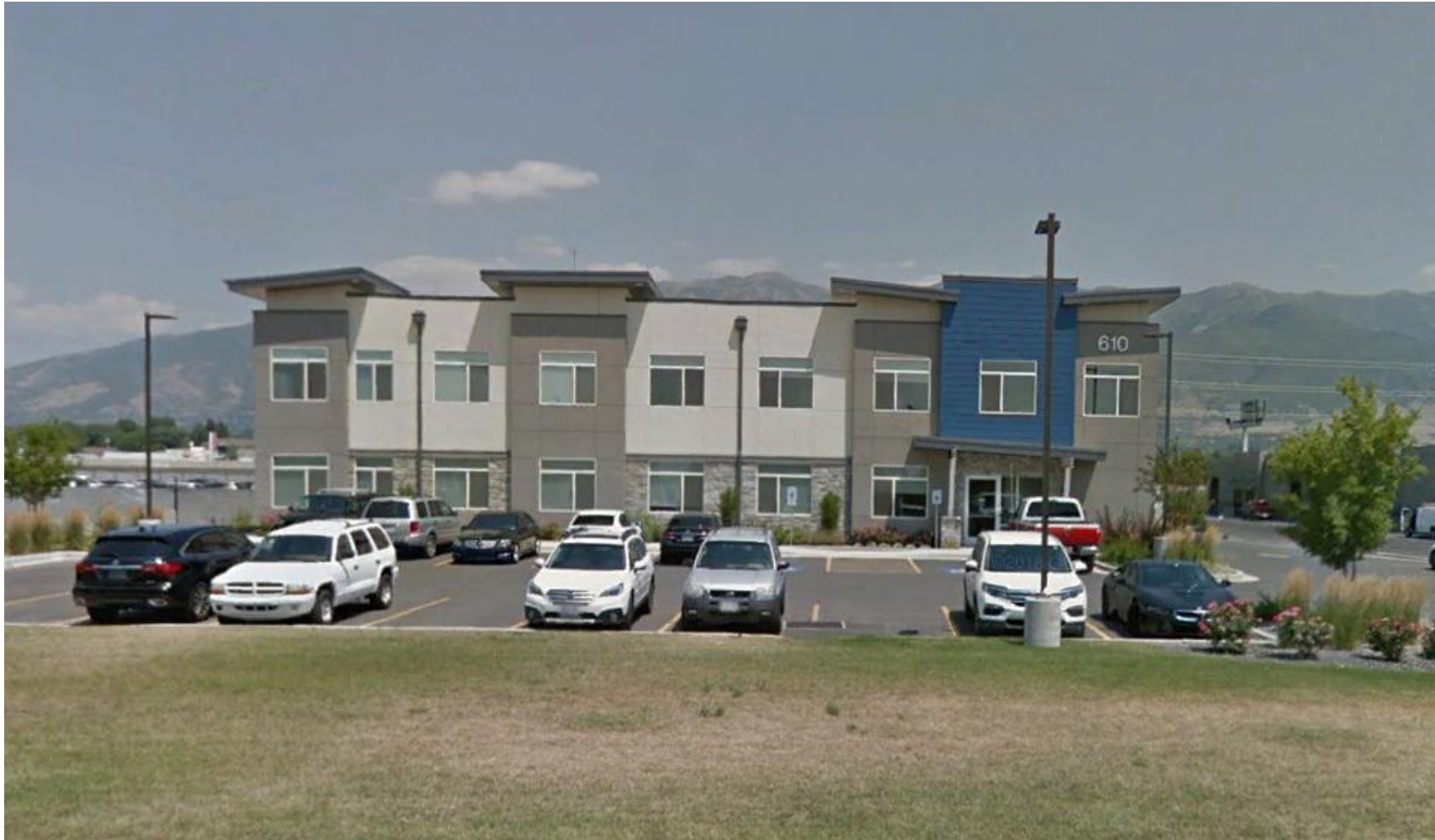
Lot 117B – Building 1 (existing)
