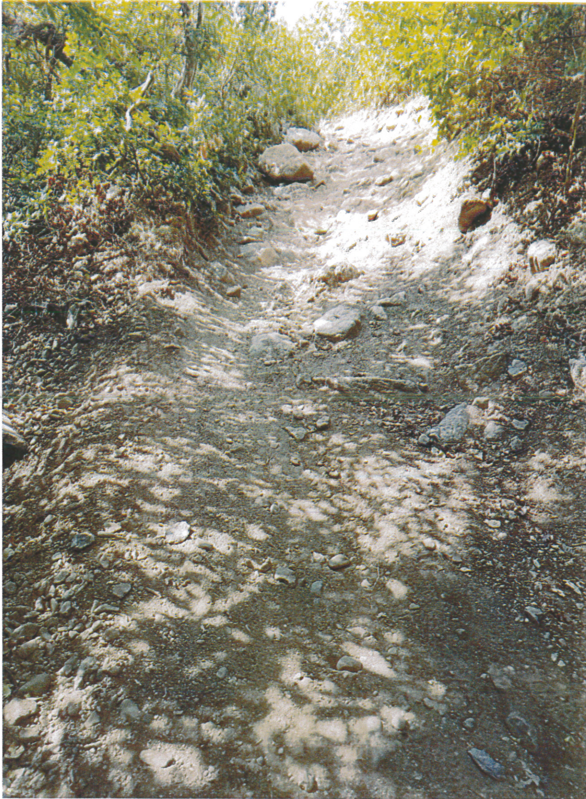
Existing trail conditions on north side of creek. (very steep)
