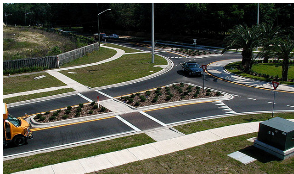
Roundabout improvements include curb ramps, marked, high visibility crosswalks, signage, and channelizers
