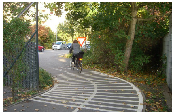
The above example shows a curve in the trail alignment combined with perpendicular pavement markings that visually and tactilely slow trail users before the intersection.
